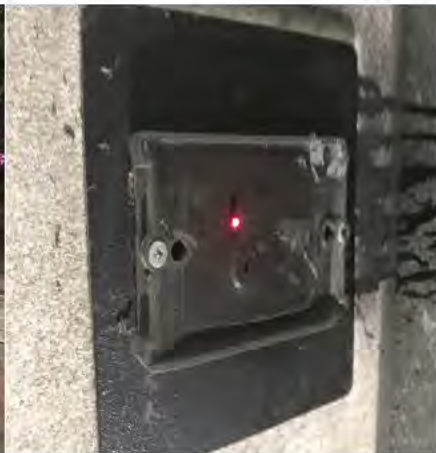
Hatfield - Burned sally port Card Reader
