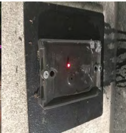
Hatfield - Burned sally port Card Reader
