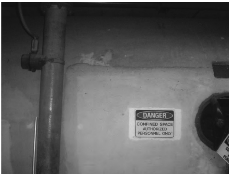
Water Tank Insulation Sample Penthouse - 12A
