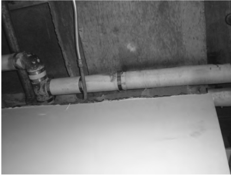
Pipe Insulation, Air Cell Sample 1 - 48A
