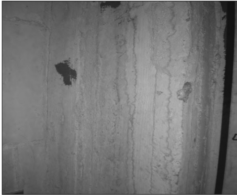
Concrete Wall Sample 1051
