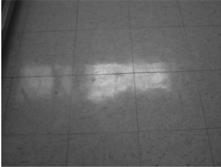
Mastic w/12"x12" Light Green Vinyl Floor Tile w/Gray Specks Sample SG - 16A
