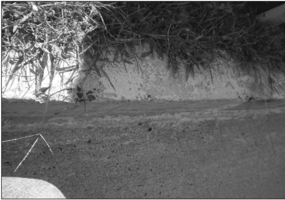
Concrete Curb Exterior Sample 1955
