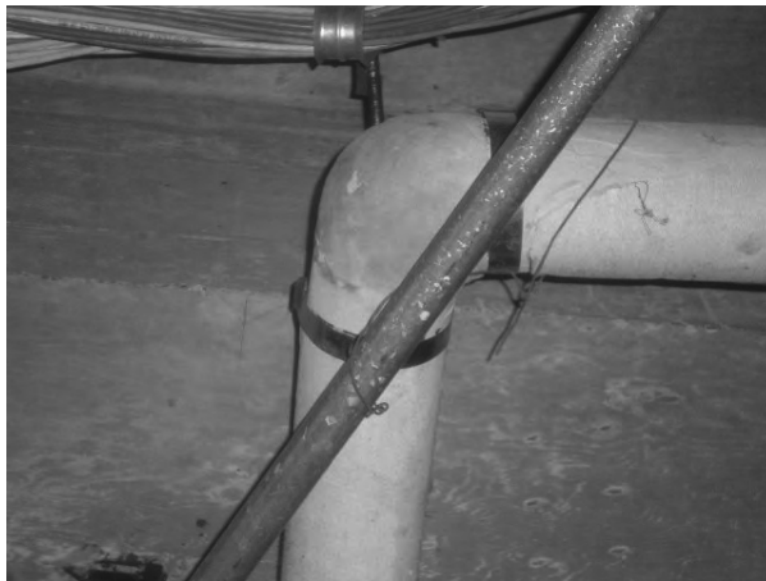
Pipe Insulation Sample G - 63A
