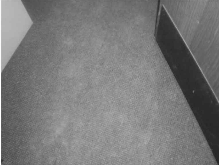
Mastic w/9"x9" Black Vinyl Floor Tile (below carpet) Sample 1 - 71A
