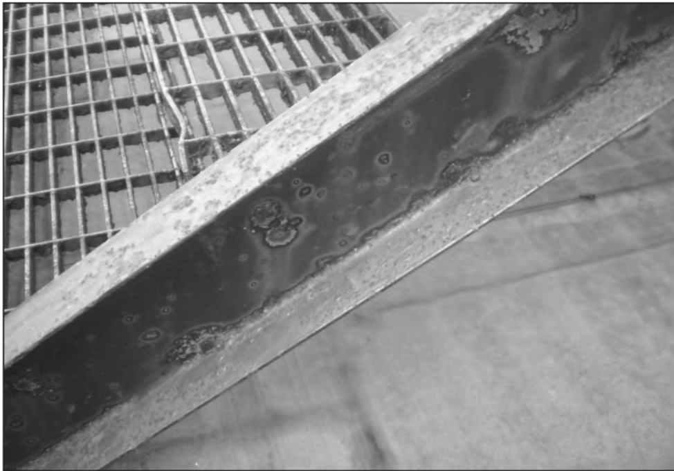
Metal Stair Stringer Exterior Sample 1978
