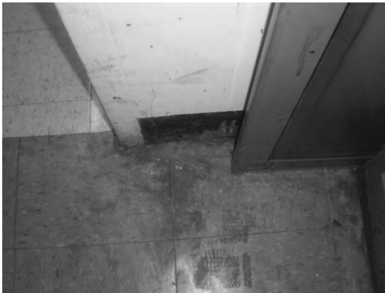
Mastic w/12"x12" Light Brown Vinyl Floor Tile w/Dark Brown Specks Sample 1 - 73A
