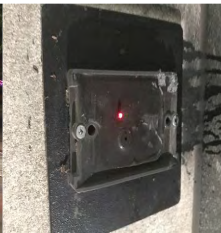
Hatfield - Burned sally port Card Reader
